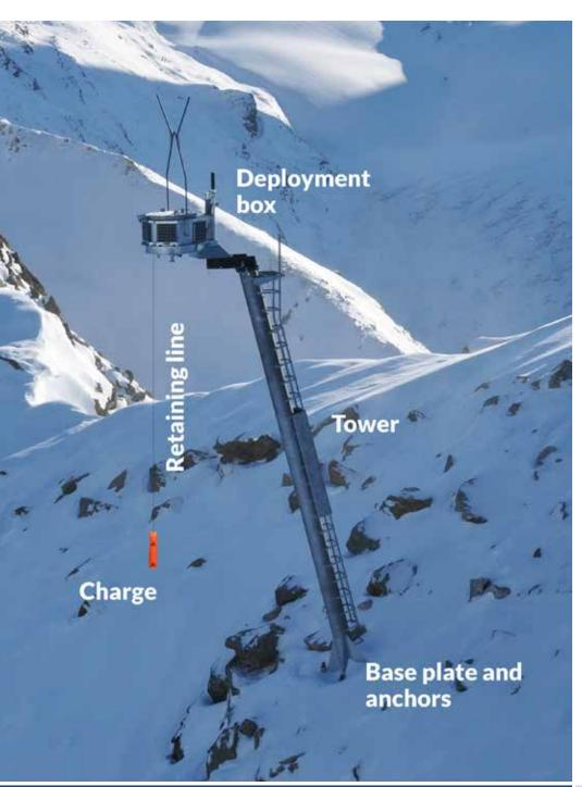
The Wyssen avalanche tower is designed to trigger avalanches prophylactically with remote-controlled blasting.
