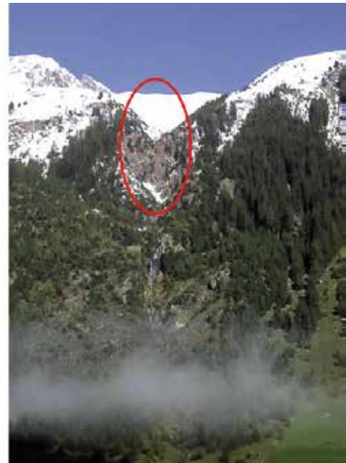
View from the radar to the opening area of the „Grosstal avalanche“. The red circle marks the surveillance area.
