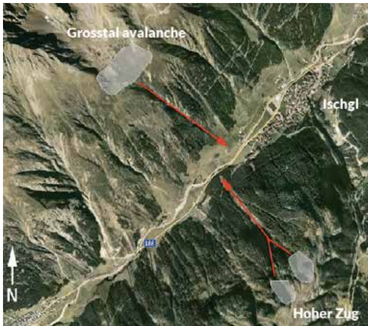
Overview „Grosstal-“ and „Hoher-Zug-Lawine“ with the endangered road (Google Earth)
